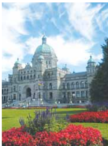
Figure 3.17 The Legislature Building in Victoria
